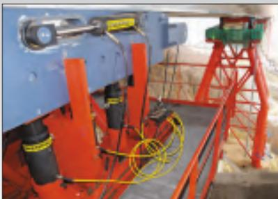
◀ Custom cylinders used for incremental bridge launching systems.
