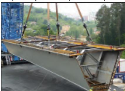
▼ SyncHoist Powerpack to operate the 4 lifting points.
