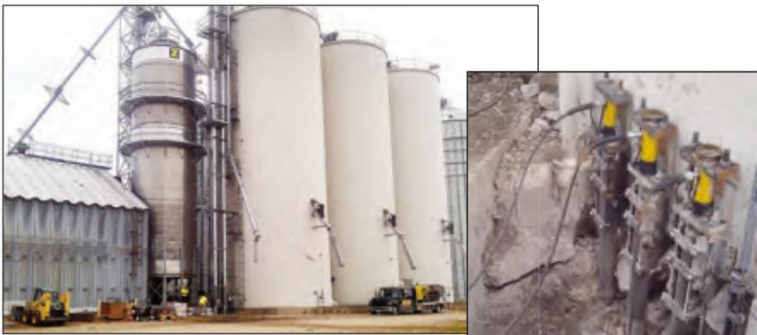
▼ RC cylinder mounting attachments greatly extend the application possibilities (available for 5, 10, 15 and 25 ton cylinders).
