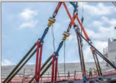
◀ Custom SyncHoist cylinders for placement of stadium roof trusses.
